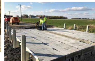
Waterproofing Bridge Decks
