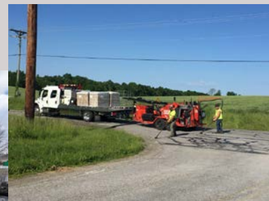
Crack Sealing
