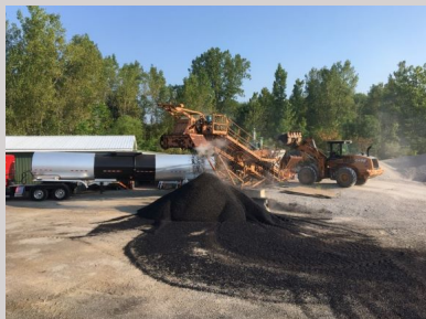
Making cold mix asphalt material
