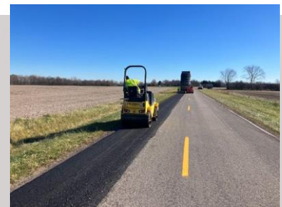
Asphalt Repairs
