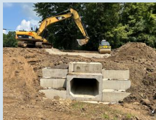
Whittlesey Road Culvert Replacement Buckeye Excavating & Construction
