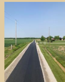
Richmond Township Willard West Improvements Gerken Paving
