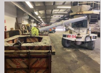
Box Culvert Construction
