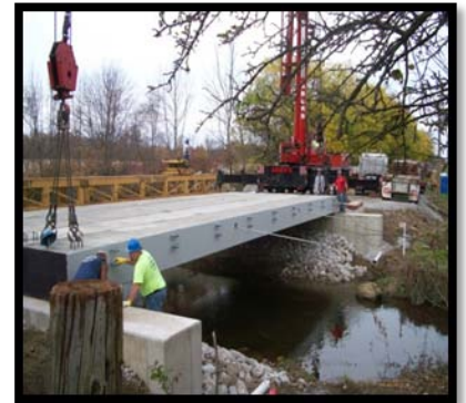
Setting beams Peru Olena / BR-164-03.62
