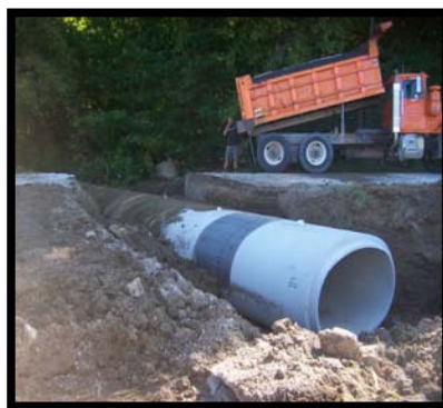
Elliptical Concrete Pipe on Fern Road
