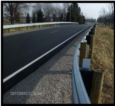
Peru Olena Road with new Guardrail
