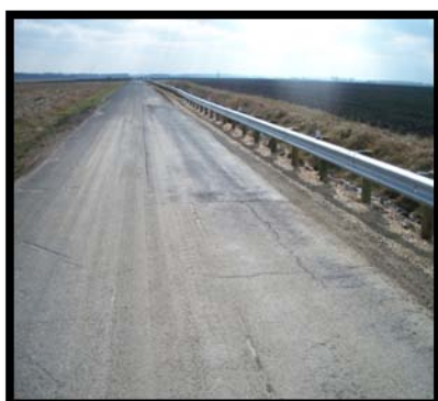
Buckingham Road Guardrail Improvements
