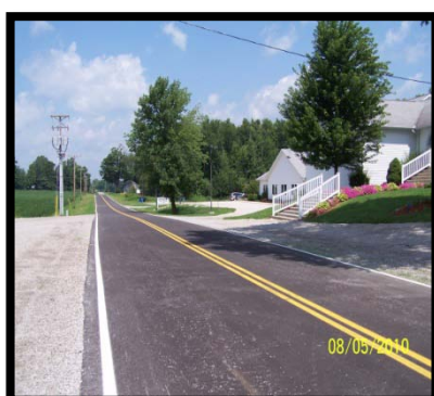
Edwards Roadway Widening & Drainage
