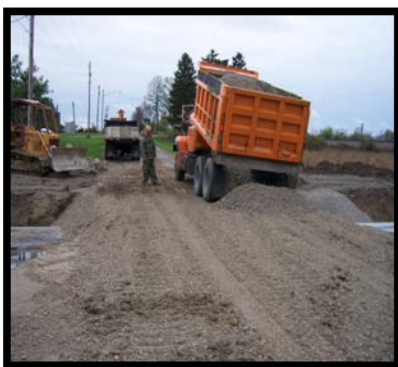
Dumping back fill on Butler Road
